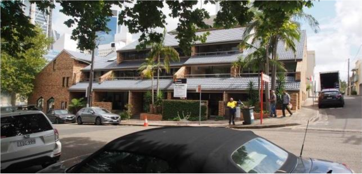
Figure 8: Site D - 263-269 Alfred Street and 4 Little Alfred Street from Whaling Road looking north (Source: Mecone)
